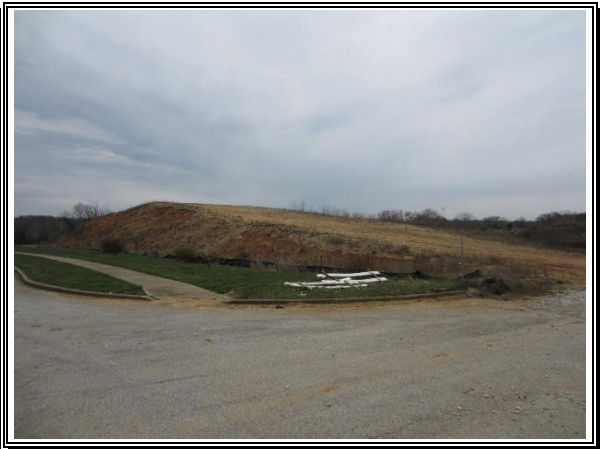
Typical Raw Ground – East of SR 46
