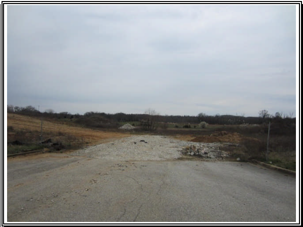
Typical Raw Ground – East of SR 46
