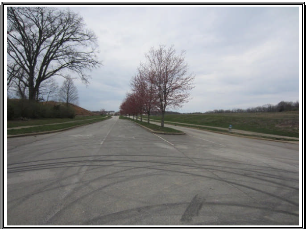
Typical Infrastructure – Stone Branch
