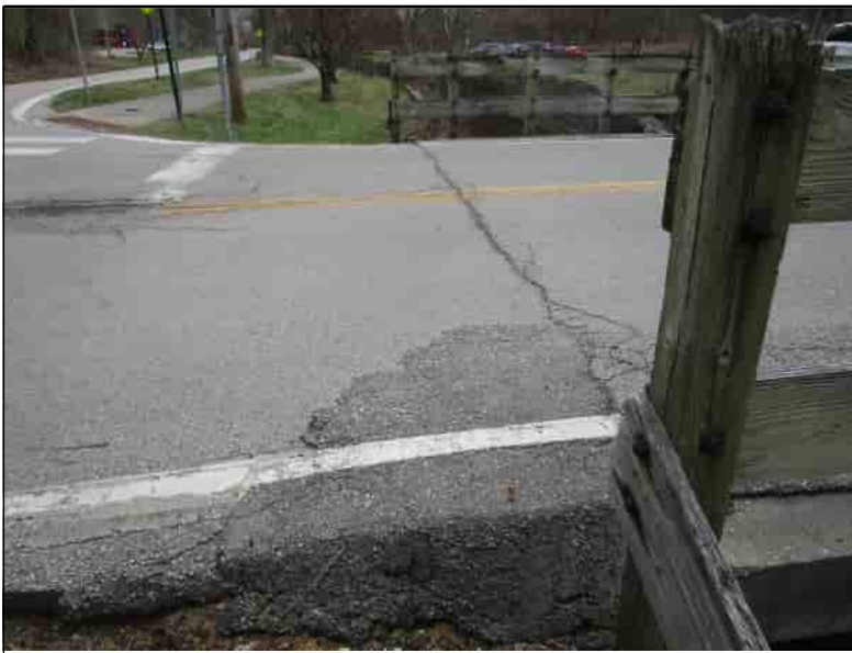
PHOTO #04: ASPHALT PATCH AT NORTHEAST CORNER
