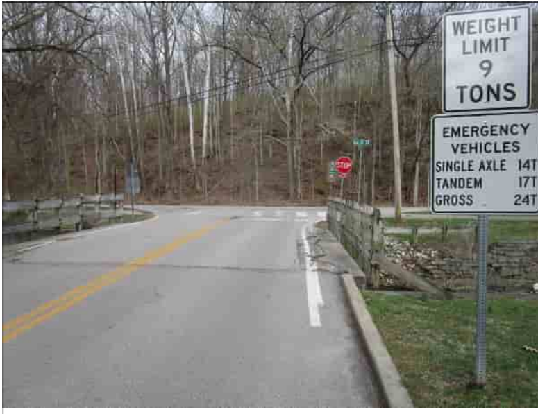
PHOTO #07: APPROACH LOOKING EAST LOAD POSTING
