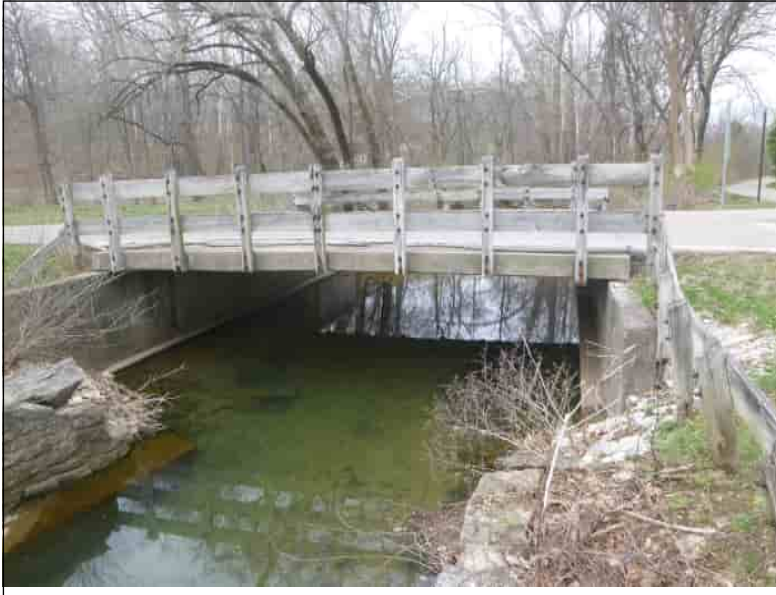
PHOTO #03: ELEVATION LOOKING NORTH
