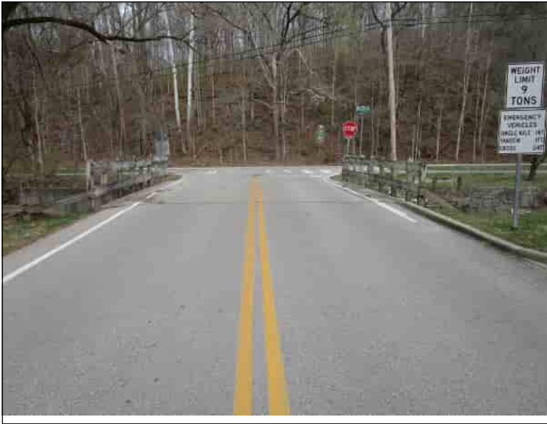
PHOTO #01: APPROACH LOOKING EAST
