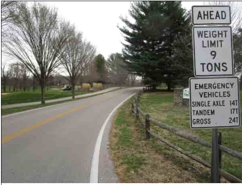
PHOTO #09: APPROACH LOOKING EAST ADVANCE LOAD POSTING
