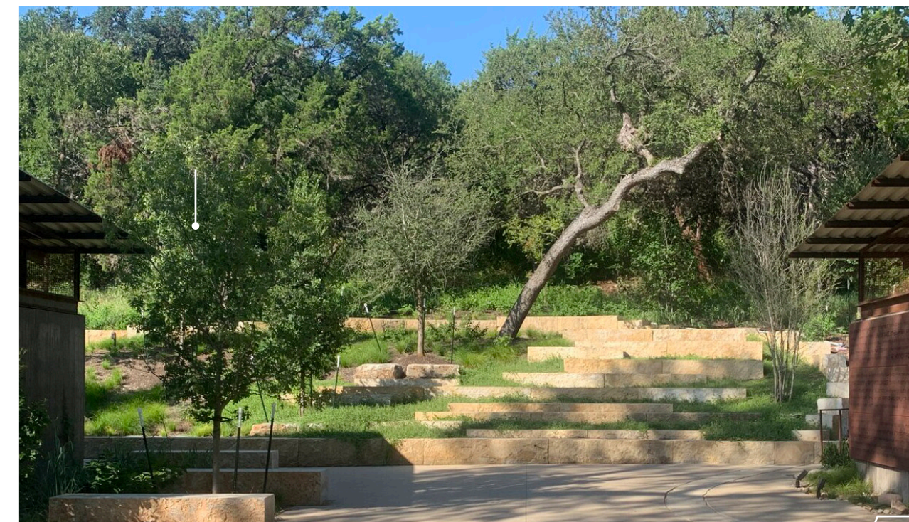
HILLSIDE TERRACING WITH STONE BLOCK
